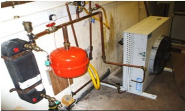
Fig. 3 Shows the connections of the heat exchanger, water pump, heat rejection fan and expansion valve.
